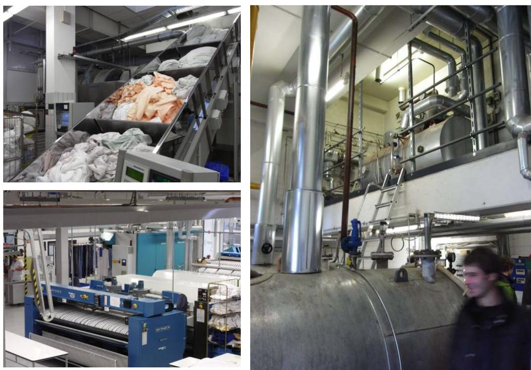
Picture. 3: Washing plant of the laundry, (left side top), ironing machine (left side bottom) and steam boiler room (right) with steam boiler (front) and feed water tank (upper floor).
