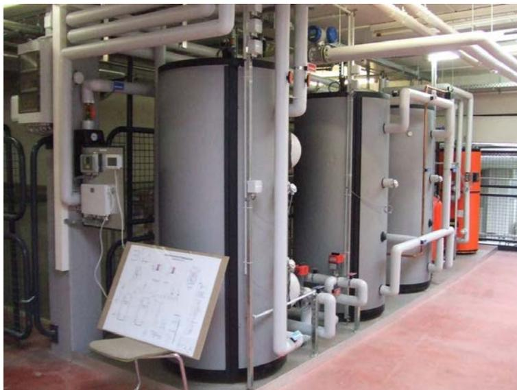
Picture. 2: Buffer storages of the solar thermal system with control unit and piping. In the front is the primary storage, in the middle the two secondary storages and in the background (orange) the buffer storage to supply the washing machines with process water.
