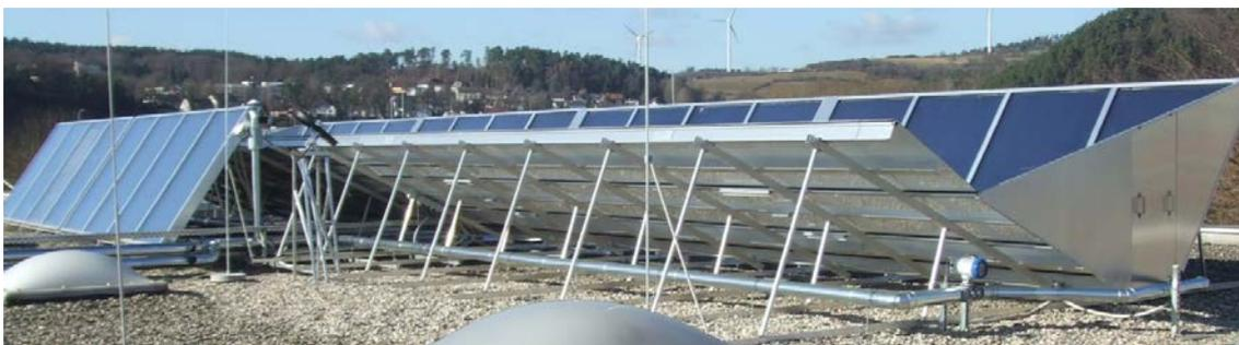
Picture 1: Collector field on the roof of the laundry. Reference flat-plate collectors (glass-foil, front) and newly developed RefleC-collectors (back), Source: S. Heß, Fraunhofer ISE
