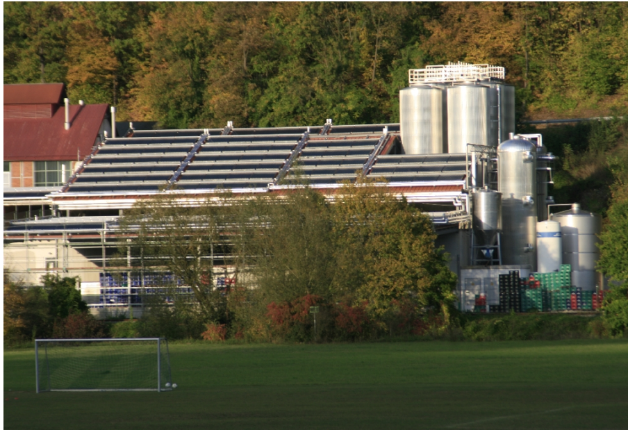
Picture 2: A part of the collector field. The two solar buffer storages are located on the right side of the building, directly beside the high storages for raw material. Source: M. Wutzler, TU Chemnitz
