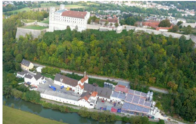
Picture 1: Location of the brewery below a castle in Eichstaett, Germany. The blue evacuated tubes are clearly visible at the right bottom side of the picture. Source: M. Wutzler, TU Chemnitz
